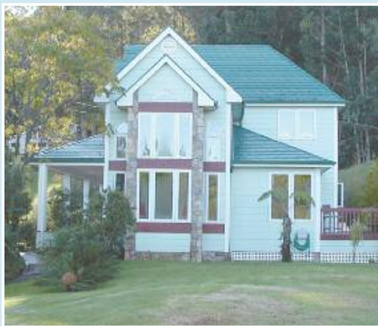
The 3 bedroom, 2 bathroom house is rich in interior and exterior detail.
